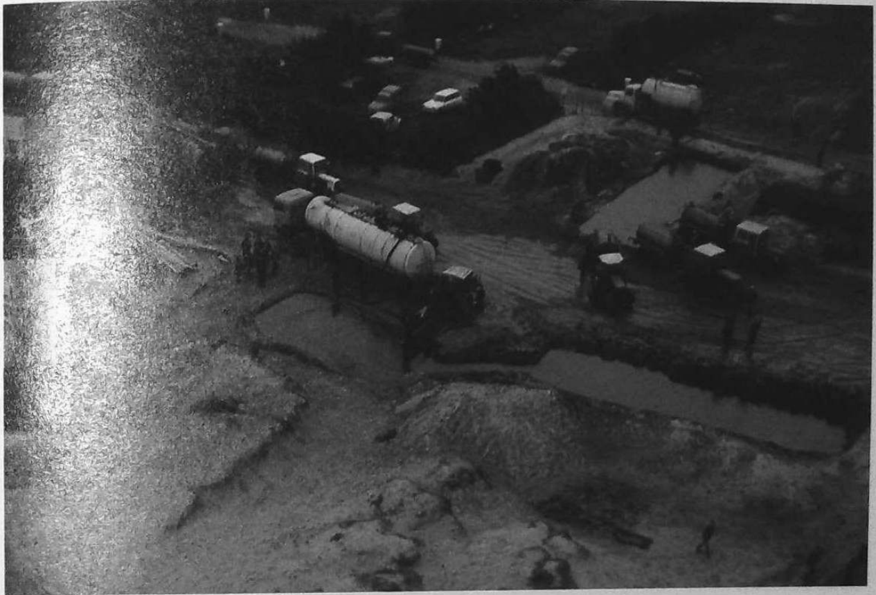
6-17. Oil/water/seaweed separation station and interim storage near Roscoff. A lesson learned from the spill is that a large interim storage has to be created, because the logistics train cannot handle the large volumes of oil removed from the water and beaches.
