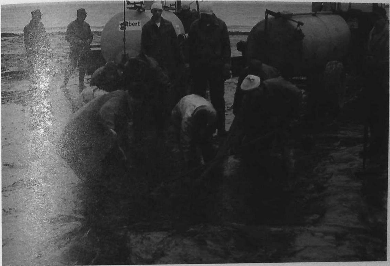
6-5. Middle dunes of the beach northeast of Portsall. Soldiers working with hand tools squeegee oil into pits where it is picked up by suction lines from two honeywagons.
