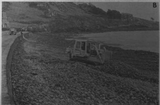
Figure 4-55. (A) Heavily oiled cobbles of station AMC-16 were pushed into furrows to aid cleaning by wave action. (B) At station F-80, a similar method of clean-up was in operation.
