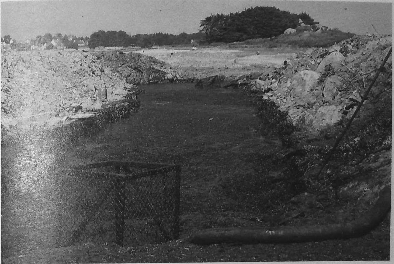
6-21. One of six ultimate disposal pits prepared in a clay area near the coastal town of Tregastel. Chemical stabilization has been considered for this material.
