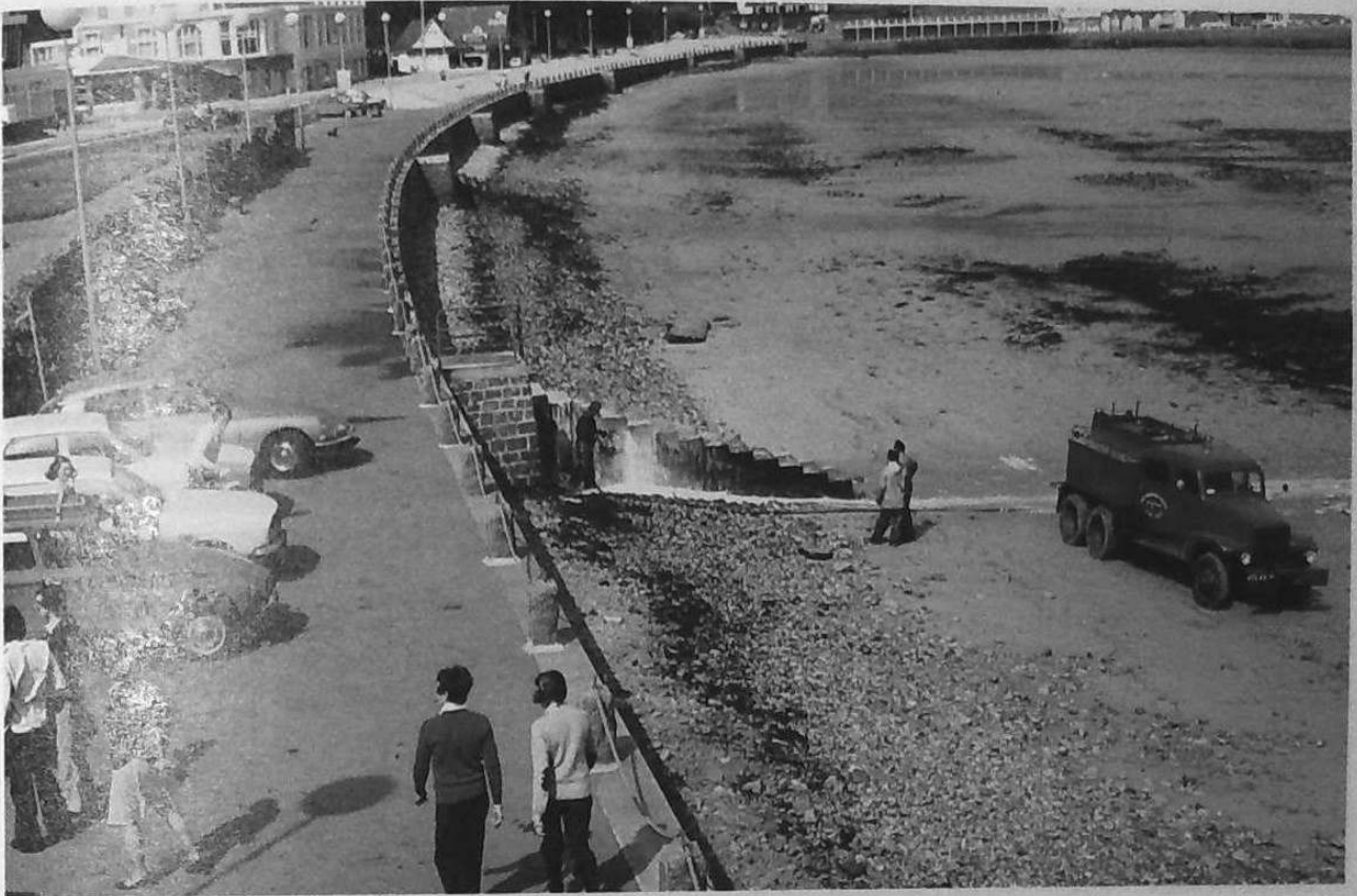
6-13. Volunteer firemen wash down steps and rocky areas with detergent solution on the beach at Perros-Guirec.
