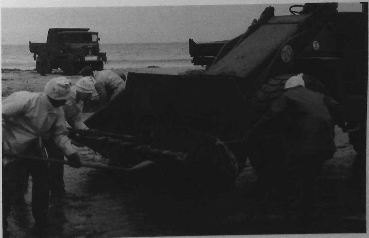
6-6. Workers scoop the oil into the loader bucket. The loader elevates it and dumps it into an Army dumptruck (shown in the background) for transport off the beach.
