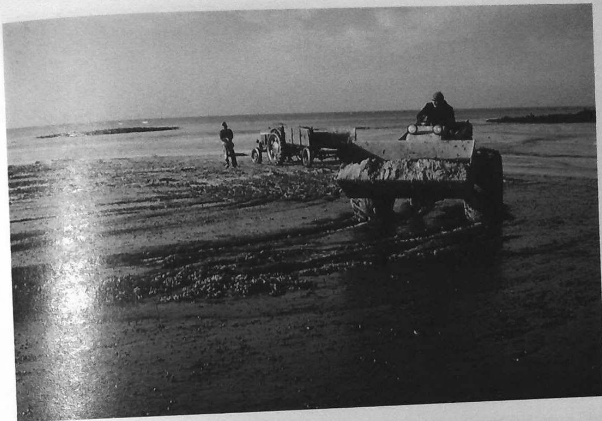
4-8. Front-end loader scooping sand at Les Dunes-West (AMC-5). In this case, a considerable amount of sand is being removed from the beach, a practice that should be avoided if at all possible. (31 March 1978)
