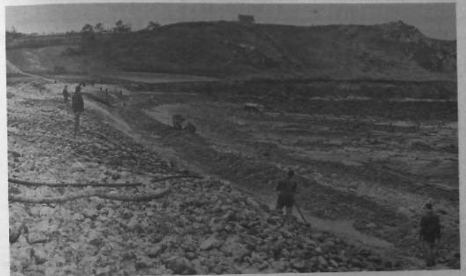
Figure 4-50. Oil clean-up at the cobble beach at station F-95 on April 27. A tractor created the runoff trench at the foot of the beach. High pressure water helped remove the deeply penetrated oil from the cobbles. The method is sound from a coastal geomorphic standpoint since beach sediment is not removed. Reworking by waves will re-establish the normal beach profile.
