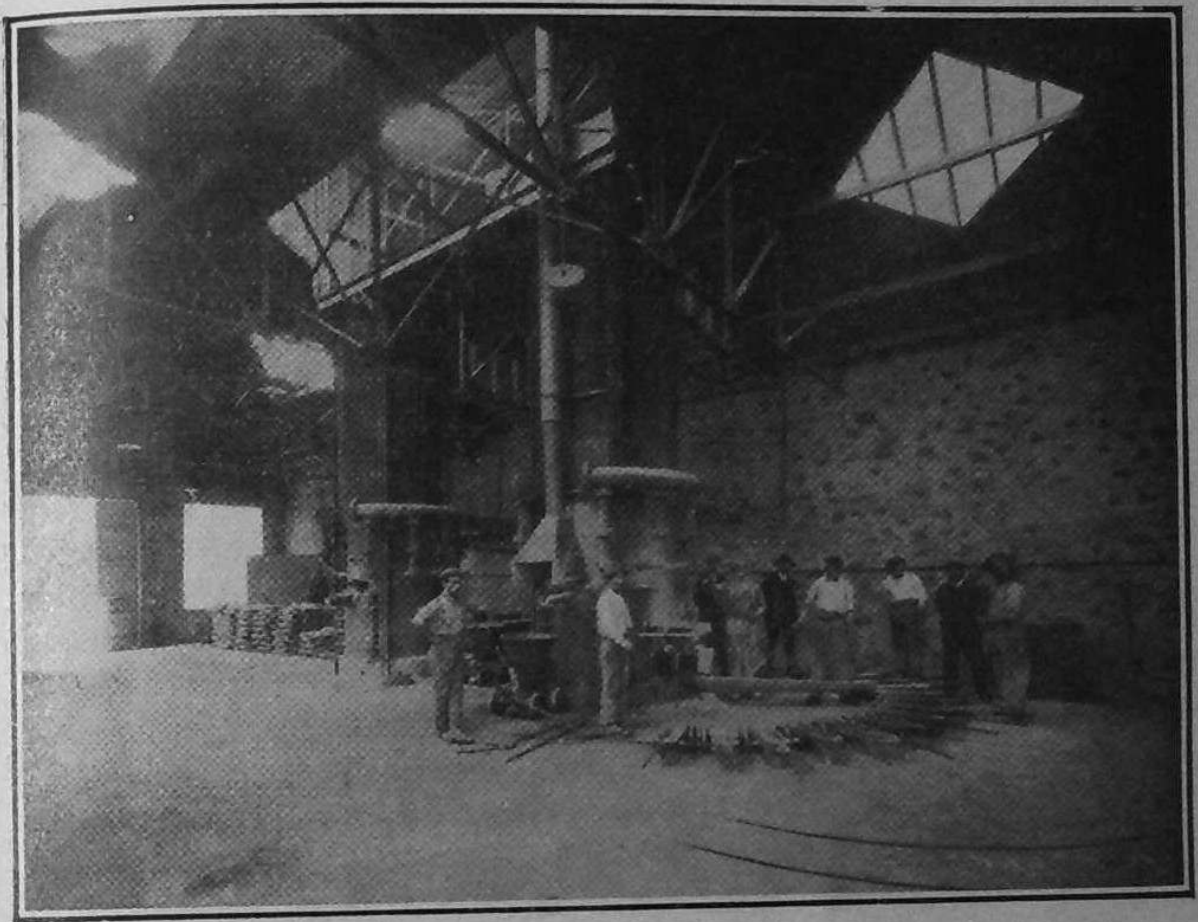
Fonderies de Saint-Brieuc. — Water-Jackets.
