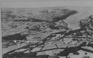
Aerial View of Menai Straits and Anglesey
