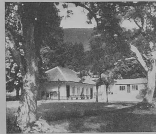
Llanerby-y-Moel, Dolcoed Wells, Pump House
