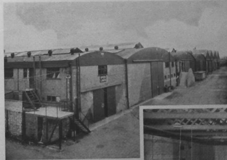
The Caerphilly factory of Welsh Metal Industries Ltd.
