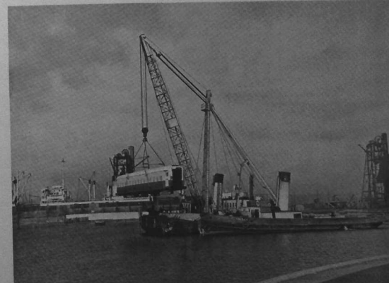
One of a Consignment of Railway Coaches for the Iraqi State Railways being shipped by floating crane. Note the Lifting Block.
