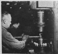
Assembling and Peening over of ball in upper links of Ferguson tractor. 120 per hour.
