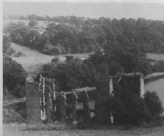
This cotton mill was built near Dornoch by Dempster of Skibo in 1790. It employed a hundred hands, and twenty houses were erected for the work people. It never made money and when it was burned down in 1808 it was abandoned
