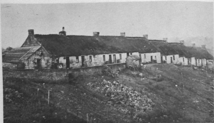
These houses at Low Quarter in Lanarkshire had turf roofs. They date from the end of the seventeenth century, and were photographed about 1890
