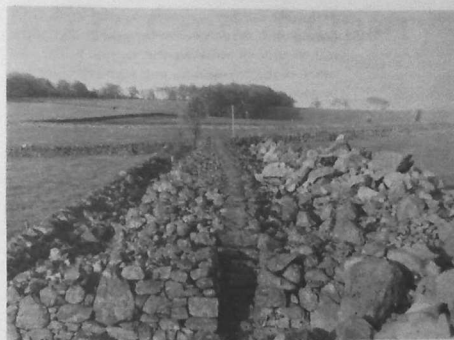
This huge dyke near Aberdeen is made entirely from the stones cleared from surrounding fields. The tenant farmers must have had a long and hard job shifting all this stone from the land
