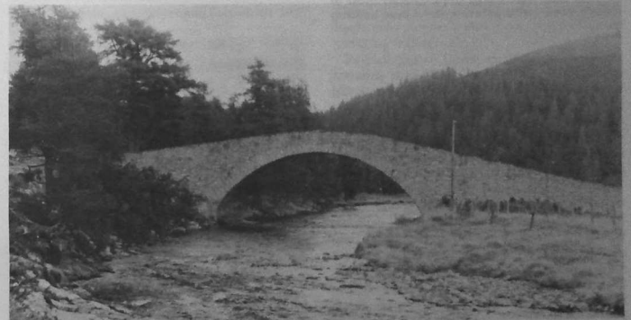
This bridge carries one of the military roads over the river Gairn in Aberdeenshire. The bridge had to be built high above the water so that it would be safe even when the river was in flood
