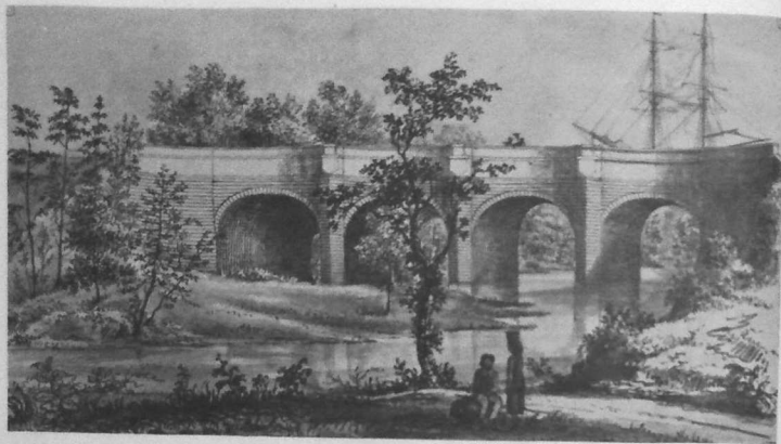
Sometimes a canal was carried over a valley by means of an aqueduct. In this print a sea-going ship is being towed over the Kelvin aqueduct on the Forth and Clyde canal
