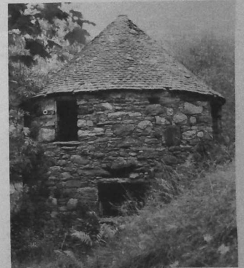
This ruined stone building was once a lint mill. It stands in a wood in the middle of the country. It was powered by a water wheel which has completely rotted away. The water which drove it was channelled from a nearby stream
