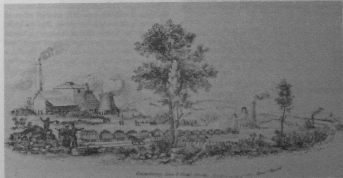
This print dates from 1831. It shows Gartsherrie ironworks in its early days, when it had only two furnaces. The Garnkirk and Glasgow railway runs across the foreground. Steam-engines were only used for long, heavy trains. Horses pulled lighter loads
