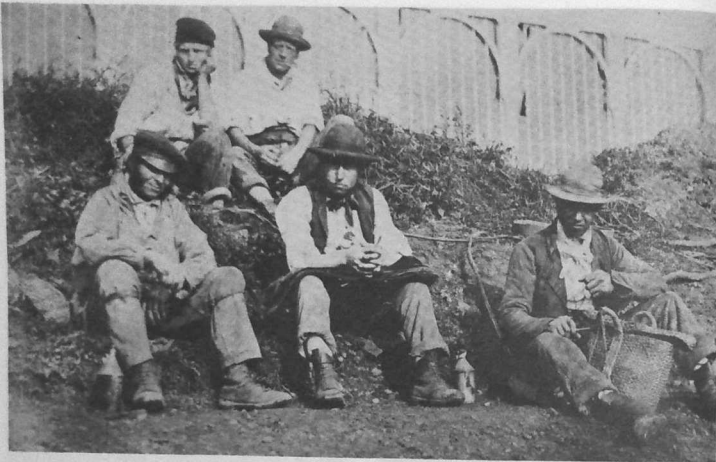
This photograph, taken in 1853, shows a group of navvies during a break from their work
