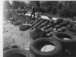
Above: Wherever possible, the Earthship uses recycled materials in its construction, the exterior walls are made with car tyres packed with earth. More earth is packed behind the tyres, and the whole grassed over. The earth acts as a heat reservoir, helping to regulate the temperature in the house.
