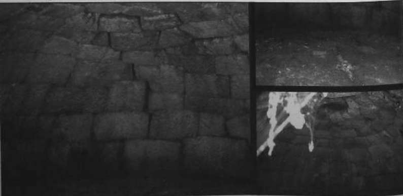
Above: Inside views of three beautifully-built bread ovens; the craftsmanship behind these old ovens, which litter the countryside, is remarkable. Shaped, tight-packed stones meant better performance, so the best quality granite blocks were used. Large, close-fitting paving slab stones make the base while evenly-sized granite blocks form the sides. Starting with large blocks at the bottom, they can be seen to graduate in size until they become quite small at the top, where they arch over to make the domed roof.
